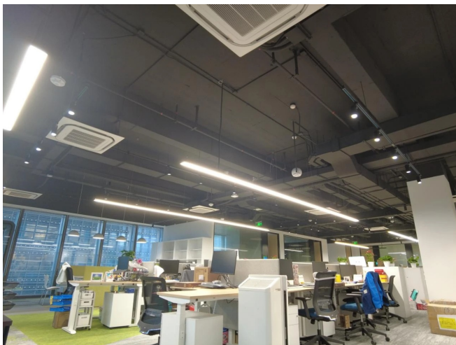
Daikin Guangzhou smart office
